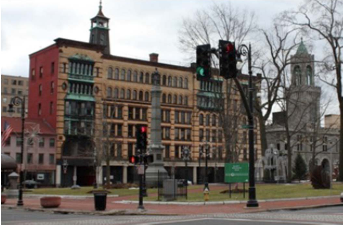
Recently Commenced 31 Elm Street Historic Redevelopment within the Target Area
