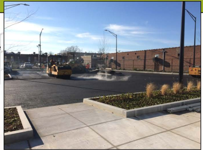
11/16 - Workers pave the employee parking lot
