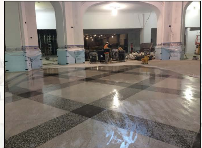
11/16 - The terrazzo floor is cleaned after repairs are made
