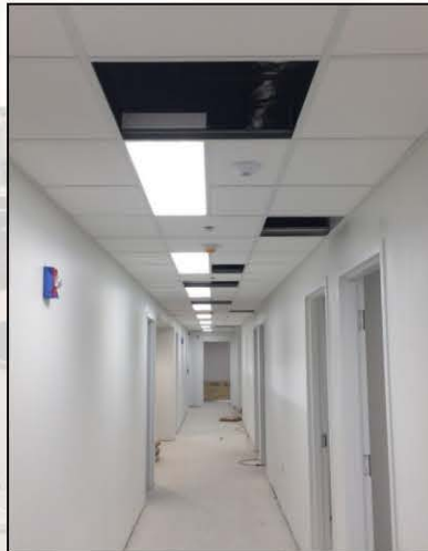
11/16 - A ground floor corridor is nearly complete
