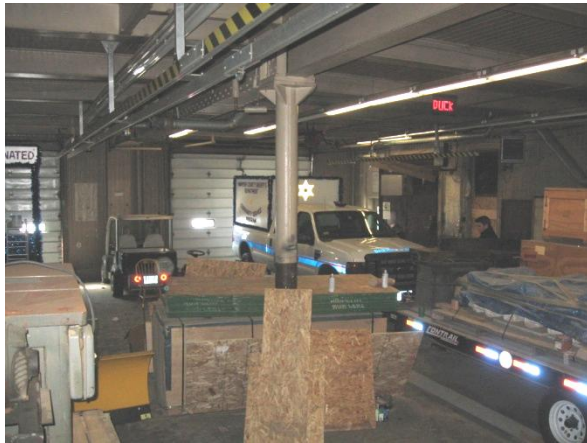
View towards the roll-up doors in the main truck garage. At least one column must remain.
