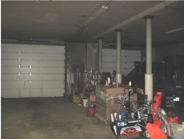
Ground floor garage space – looking towards the Oak Street roll-up doors.
