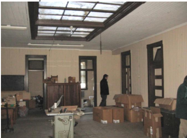
Large skylight over upstairs common room – original woodwork and partitions are largely intact.
