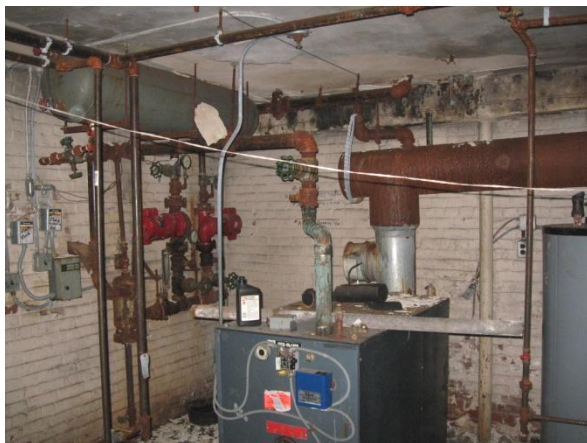
New mechanical systems were installed in the 1960's. Most of the basement was walled off and filled in.
