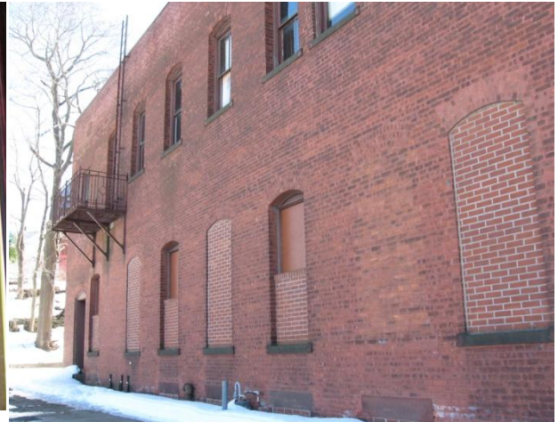
Some windows are blocked, but the infill is easily removed.
