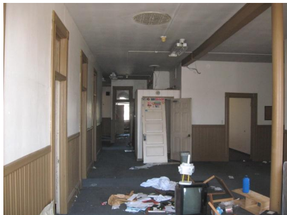
Standing in the firemen's common room, looking towards the rear.
