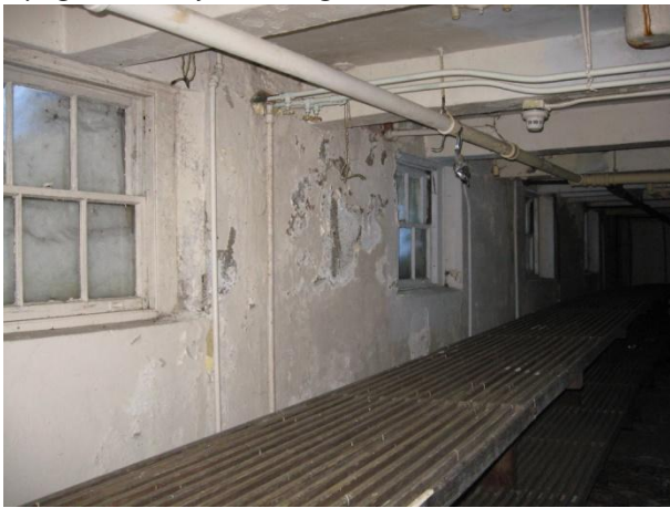
Light wells at basement provided ventilation to the hose drying area and kitchen/dining room.
