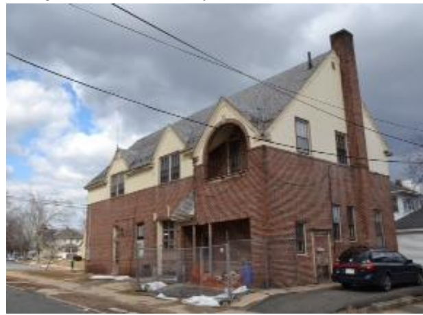
Side elevation and neighbor's driveway. Existing wood windows have aluminum storm sash.
