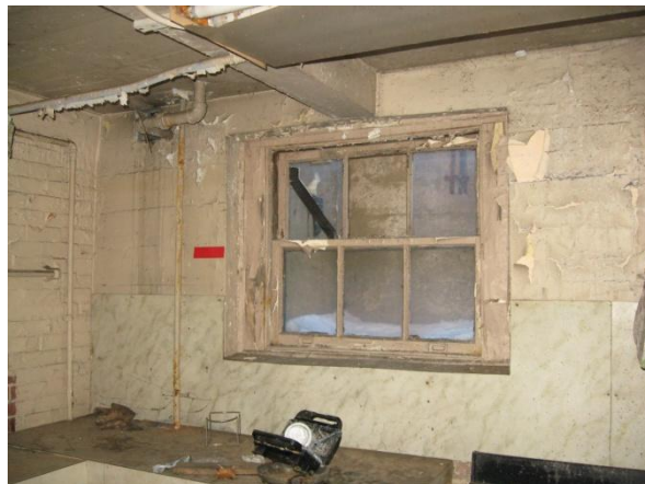
There are some unexpected touches – such as this marble wainscot in the basement kitchen/dining area.
