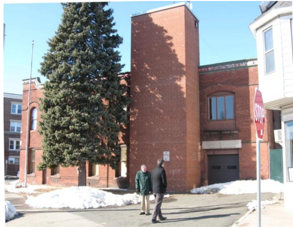
The 1960's hose tower might be re-purposed as an elevator shaft. The entry is to the left of the tower.
