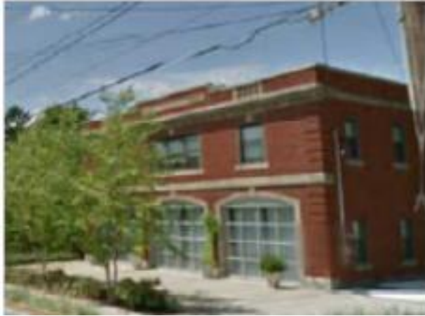
Garage doors were replaced with operable insulating glass units
