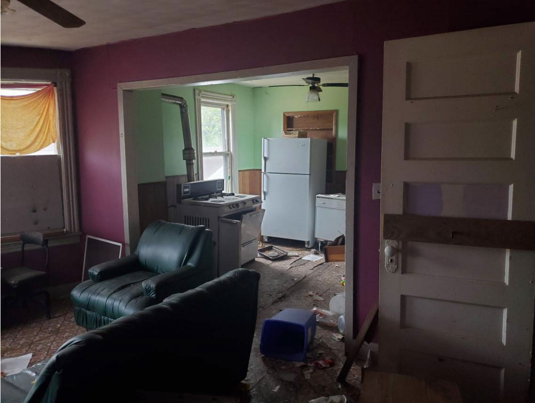
241 Main St, Indian Orchard – Representative photos of Unit 4L which is still in it's original condition. This is the only unit in the building that is not fully gutted.
