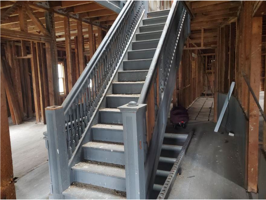
Central staircase from 2nd to 3rd floors.
