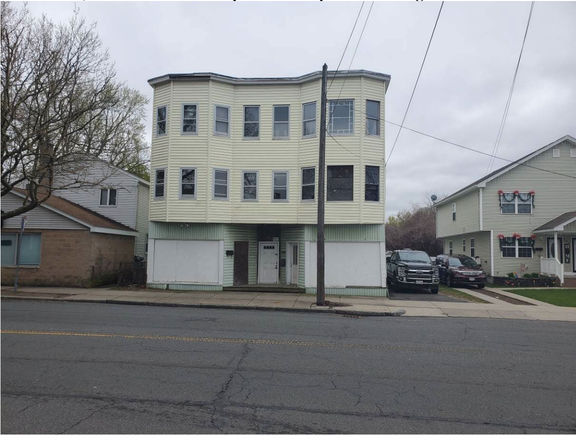
241 Main St, Indian Orchard – Representative photos showing front and rear exterior.
