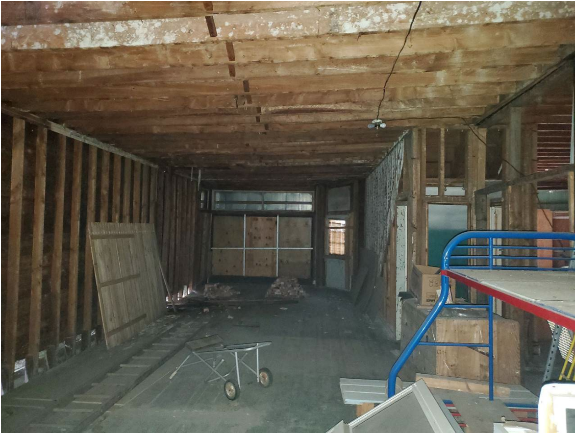
241 Main St, Indian Orchard – Representative photos of 1st floor commercial units.
