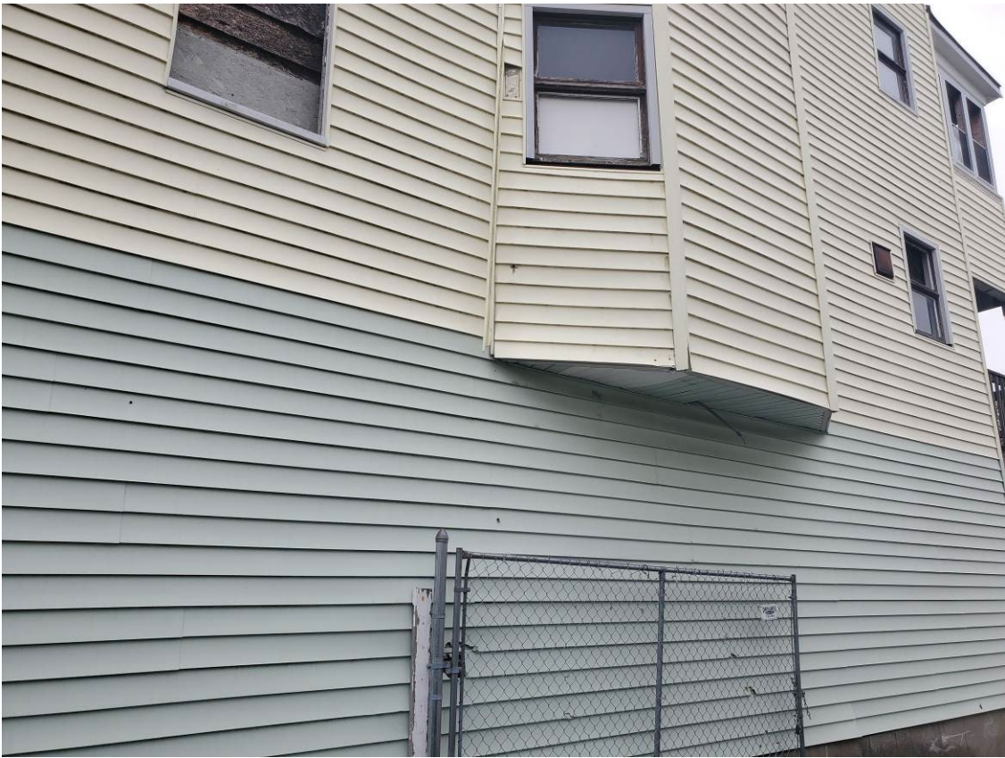
241 Main St, Indian Orchard – Representative photos showing close-up of siding.
