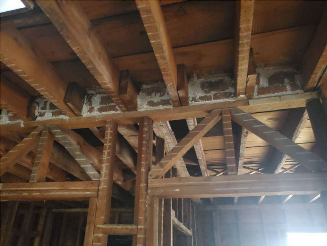
Detail of framing between 3 rd floor and roof.
