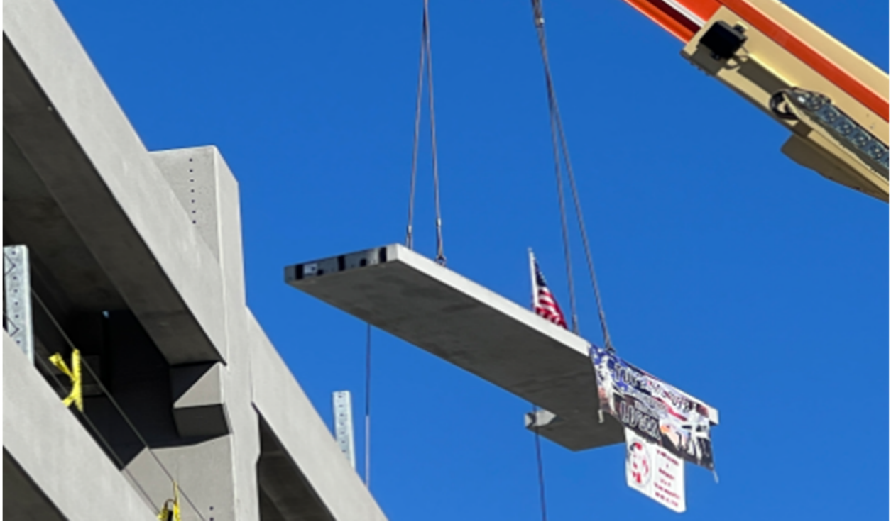
A view of the topping off of the new Civic Center garage. The $80M project will provide state-of-the-art parking and amenities.
