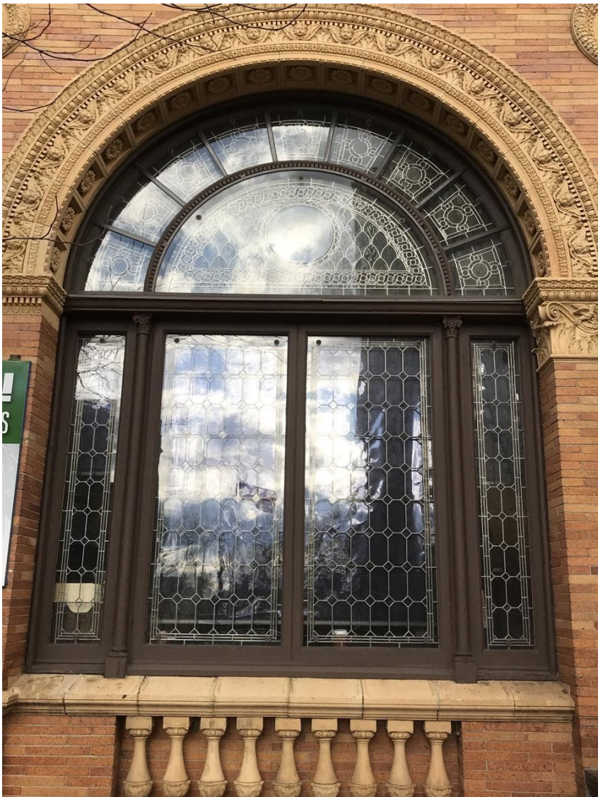
Above: Five of the eight stained glass windows proposed for restoration, located on the second floor exterior, exhibiting deterioration, and missing protective glazing.
