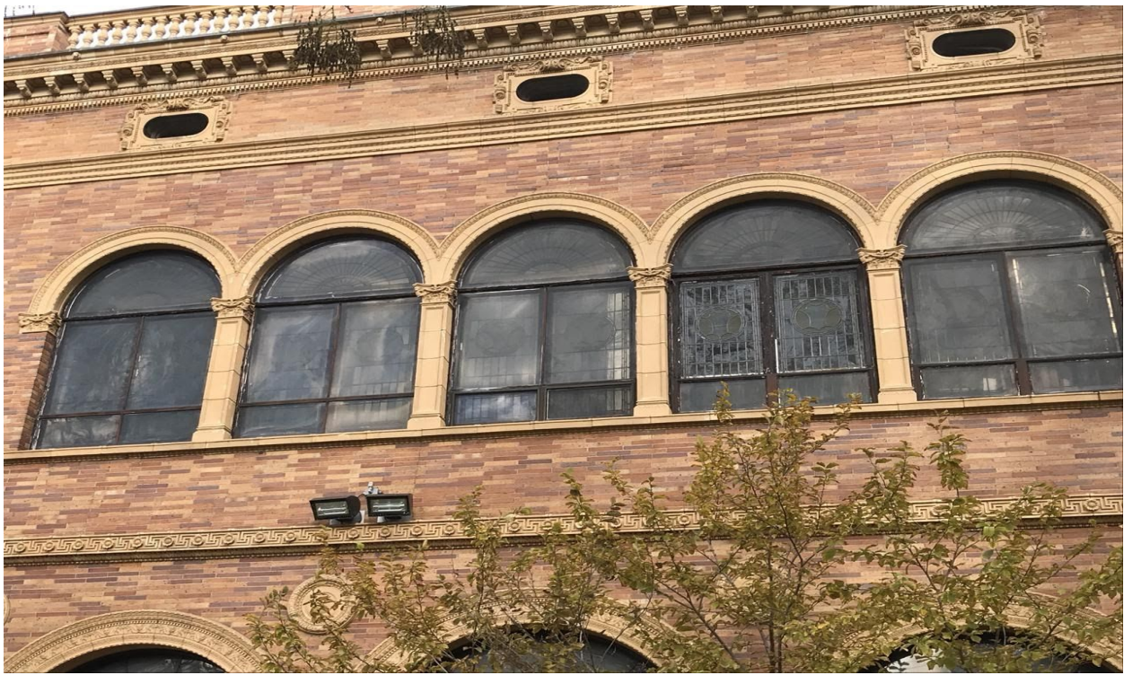
Above: Five of the eight stained glass windows proposed for restoration, located on the second floor exterior, exhibiting deterioration, and missing protective glazing.
