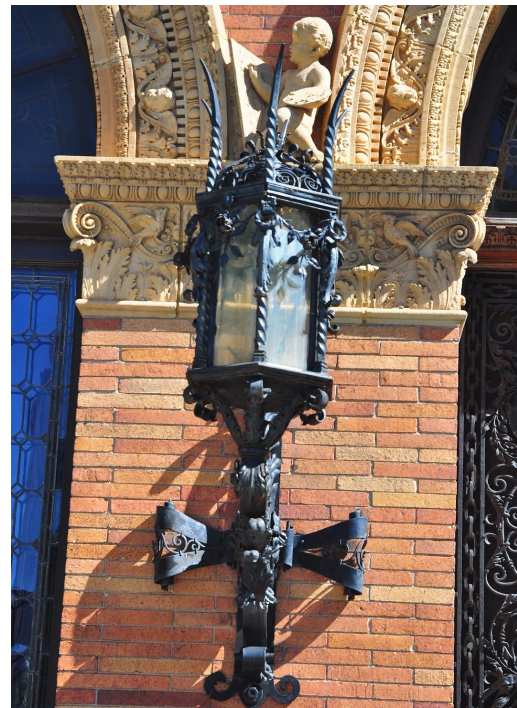
Above: loss to brownstone and masonry at front entryway. Below: loss of decorative elements and rust on sconces
