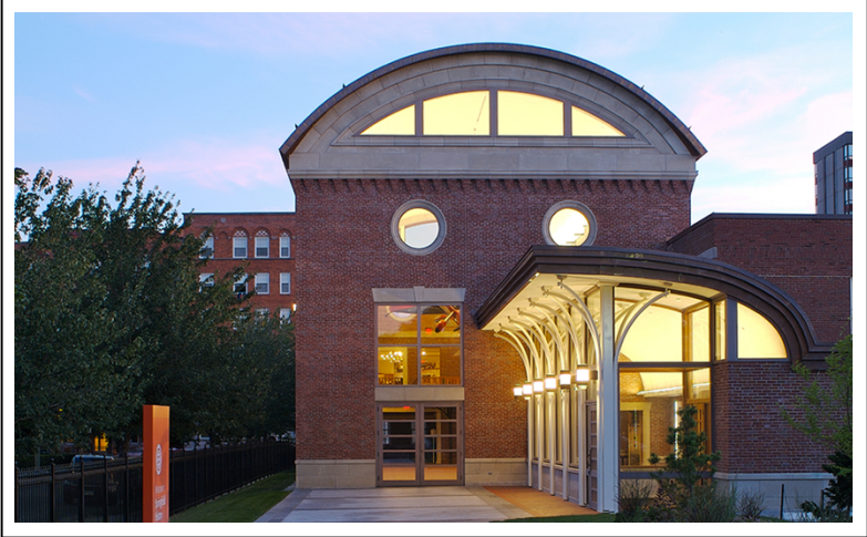
Museum of Springfield History Springfield, Massachusetts Adaptive Reuse: former office building to museum
