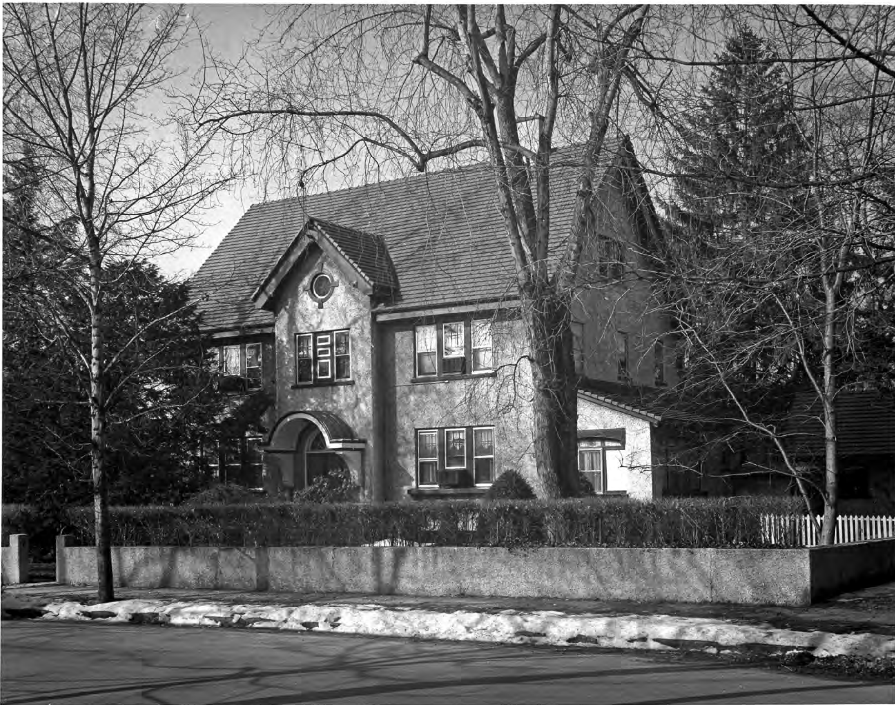
8. Looking southeast at north side Oxford Street, #6
