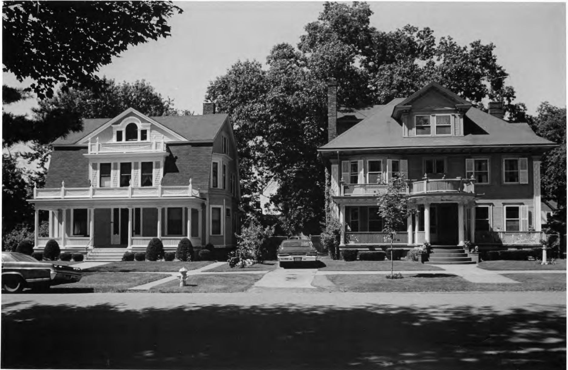
12. Looking south at west side Forest Park Avenue: #300 and #306.
