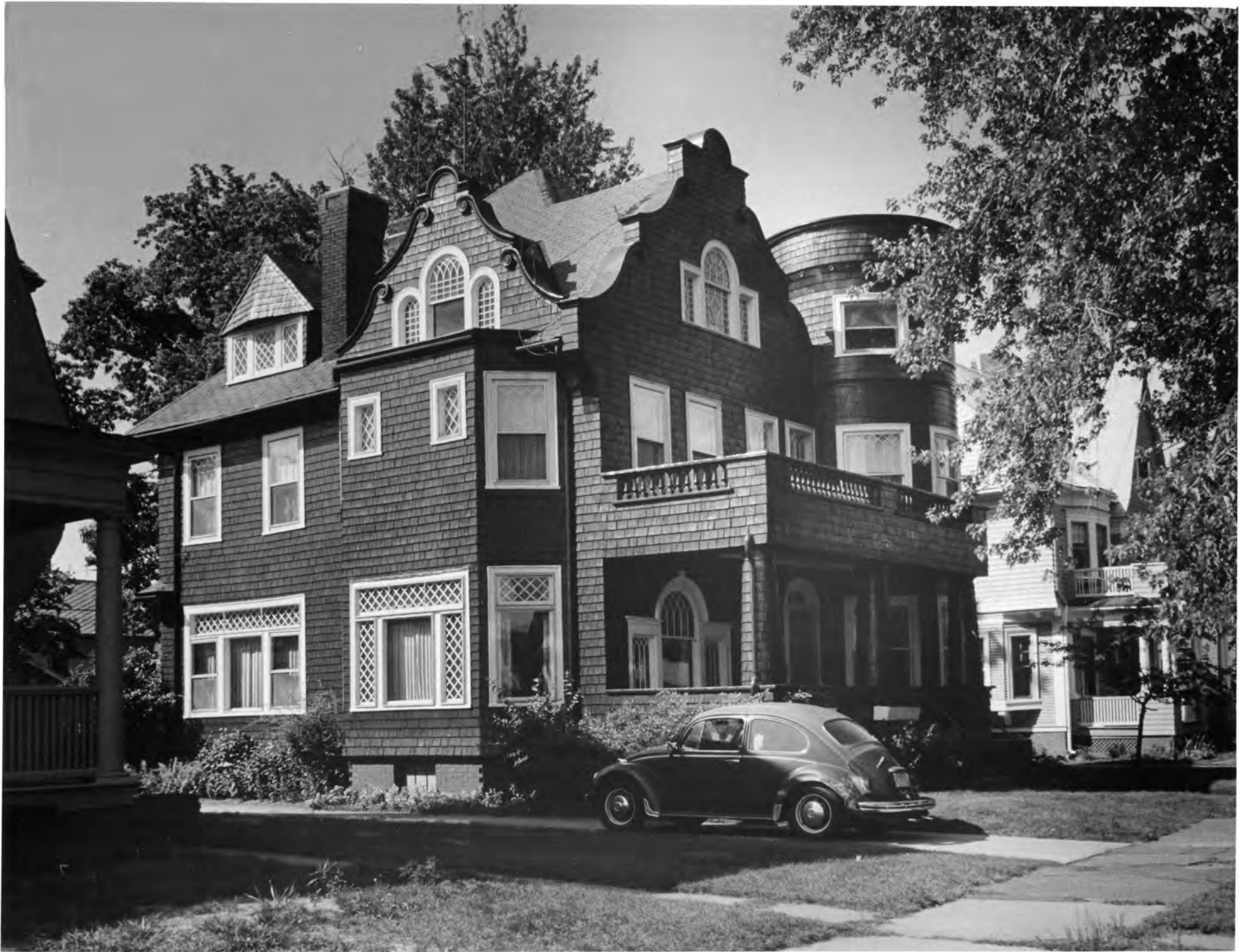
13. Looking southeast at north side Fairfield Street: #14
