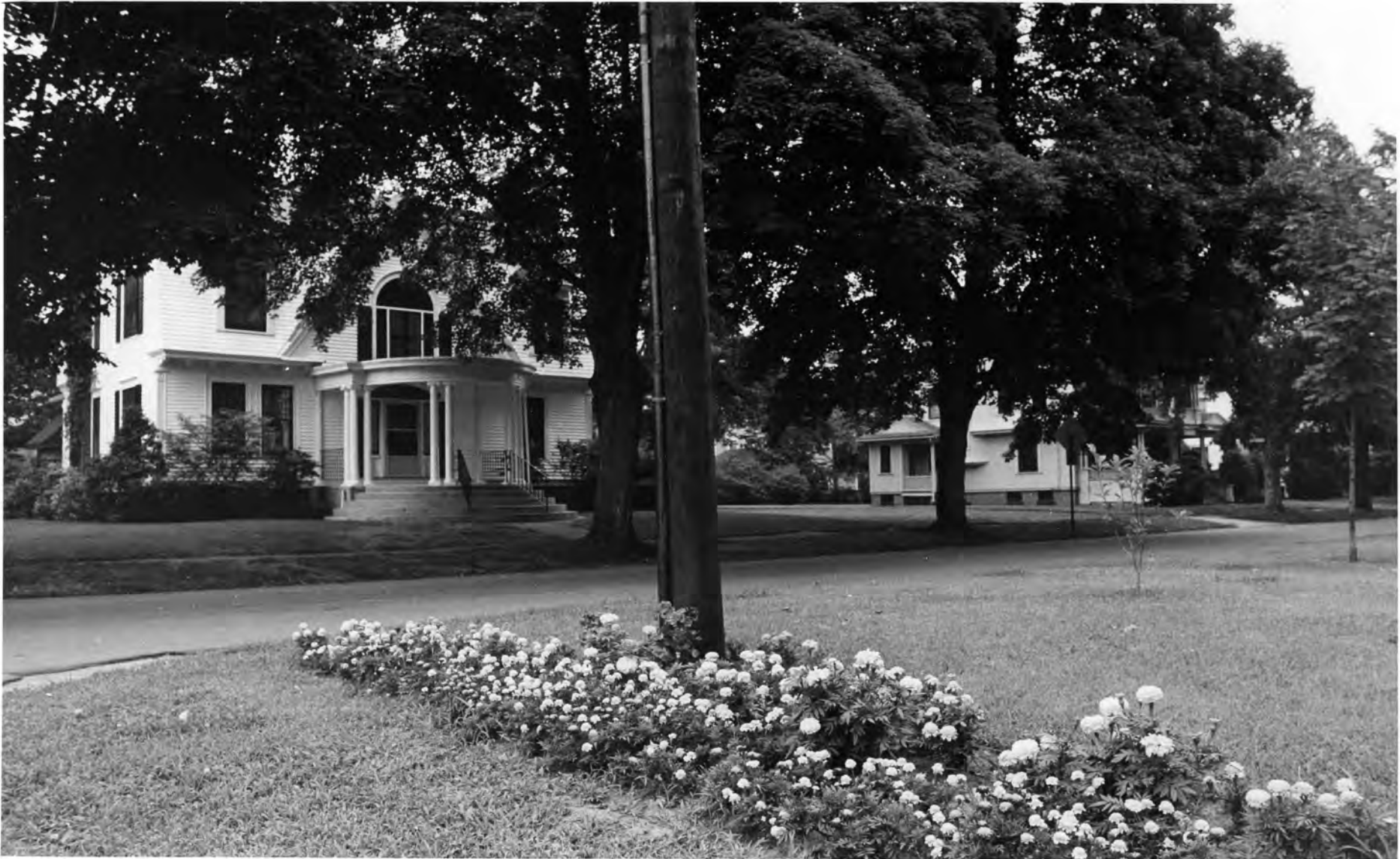
6. Looking south at east side Magnolia Terrace: #63 and #77.
