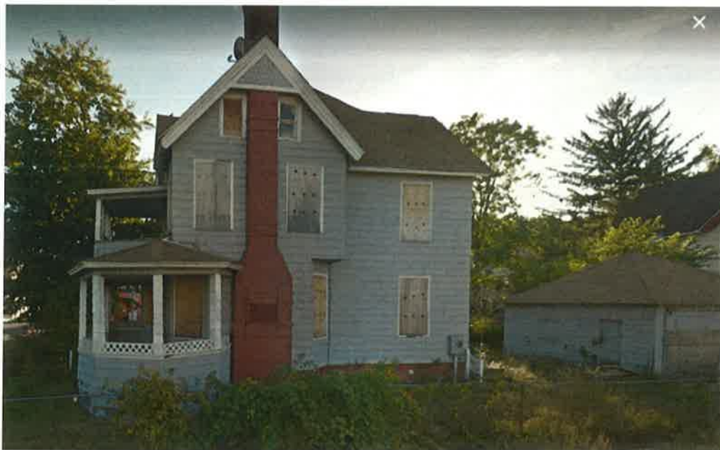
332 Bay Street at time of acquisition prior to demolition.
