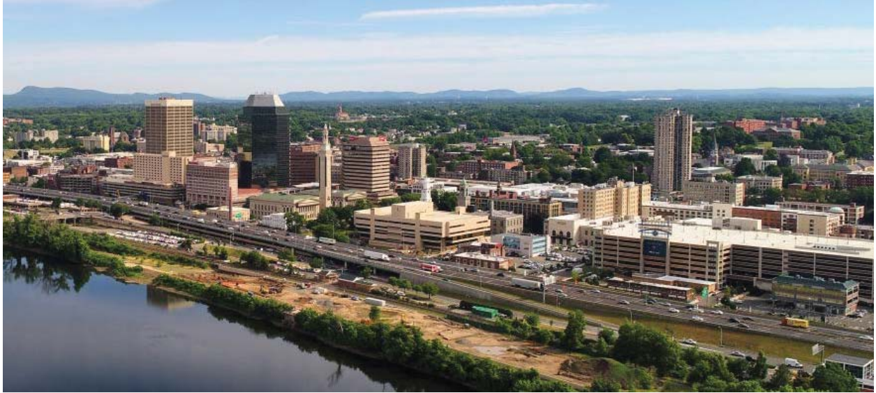
Riverfront Park, under construction 2018
