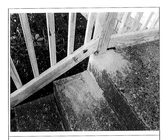
Notes: Unit 53 — Repair concrete on steps to front entry area
