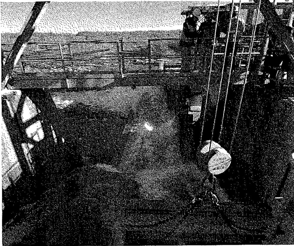
*Inspection of downstream fish passage facilities conceptually designed and computationally modeled by Alden for the Hadley Falls Hydroelectric Station on the Connecticut River*
