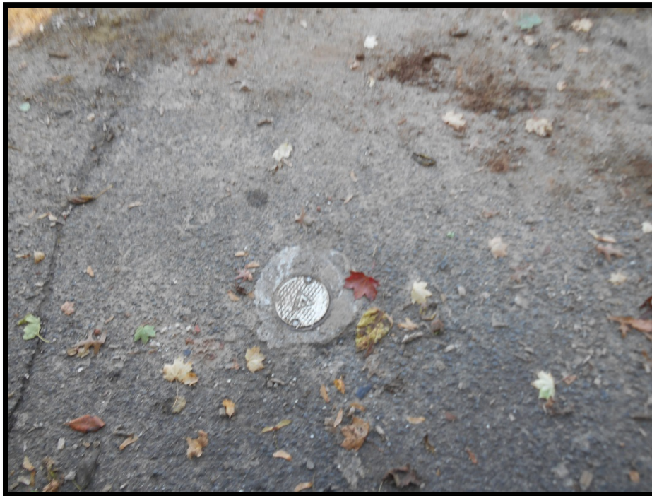
Photograph 6: View of monitoring well prior to decommissioning
