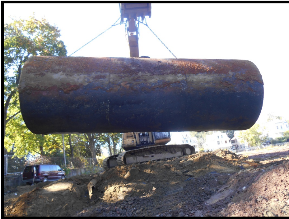
Photograph 3: View of UST side wall and bottom
