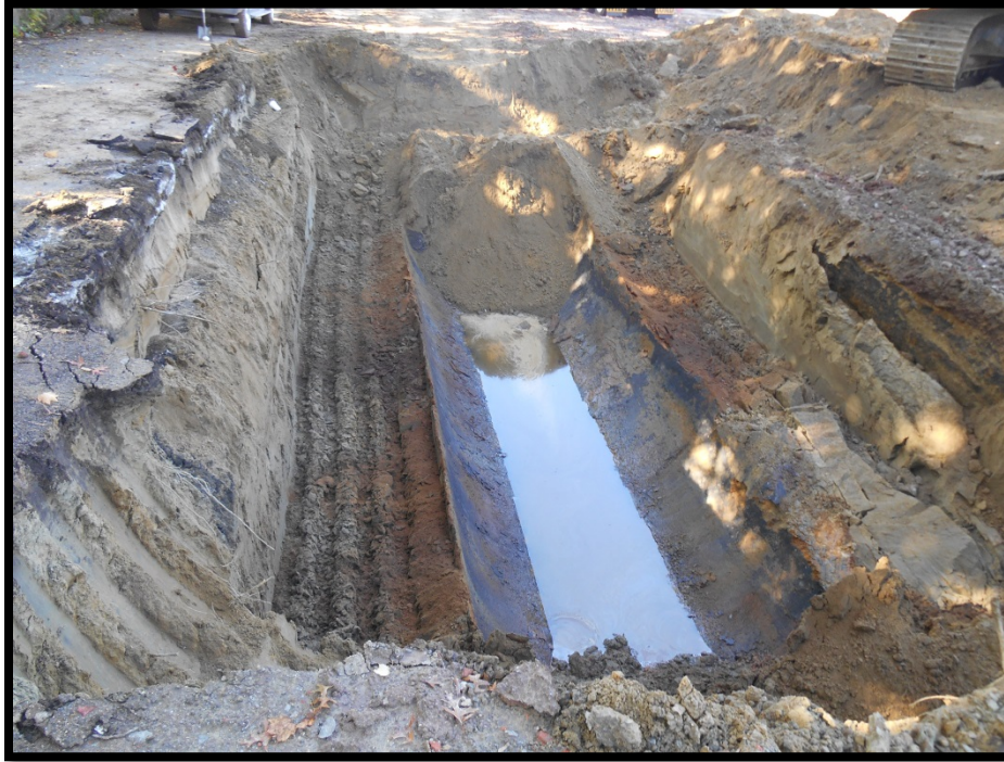
Photograph 1: Tank grave after removal
