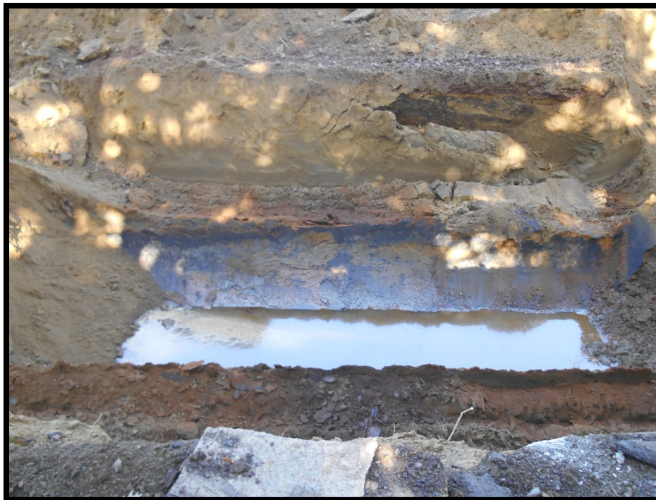
Photograph 2: Tank grave side wall
