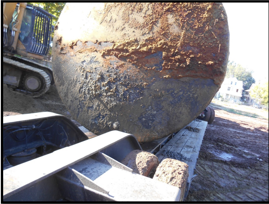
Photograph 5: View of UST end wall
