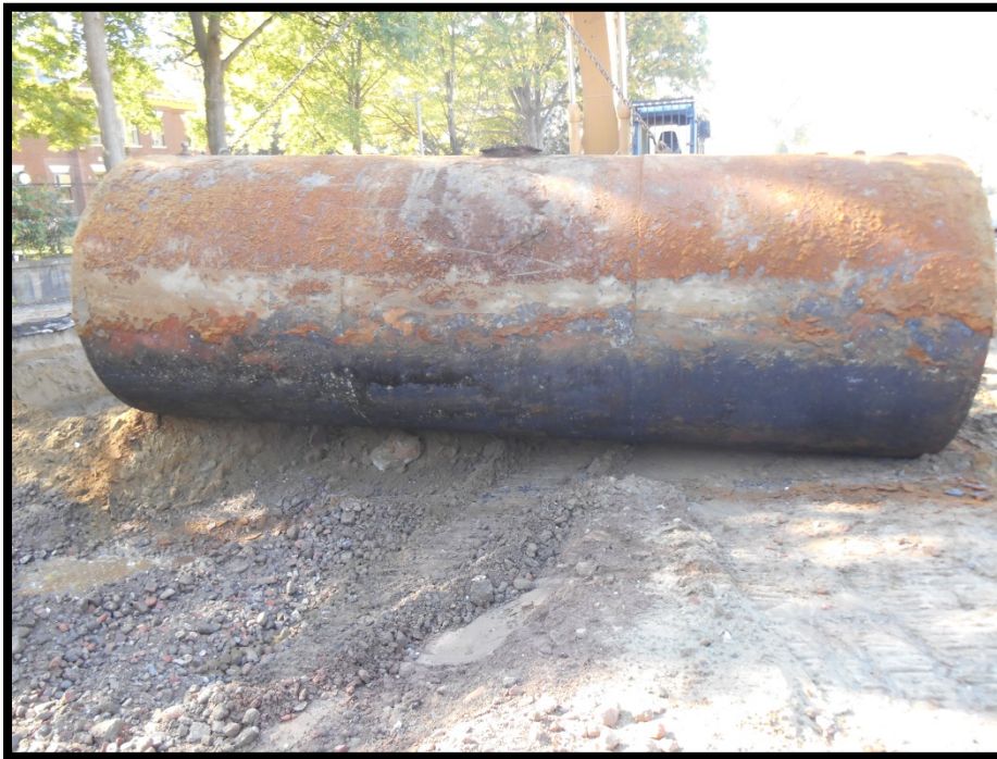
Photograph 4: View of UST side wall
