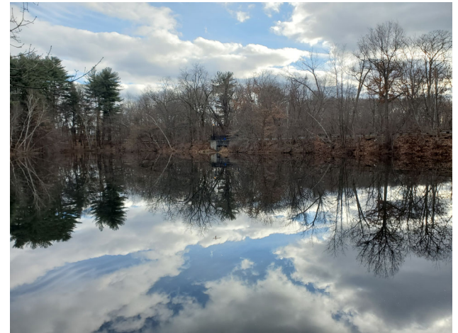
View of Upper Van Horn Reservoir facing downstream with dam and concrete spillway in background
