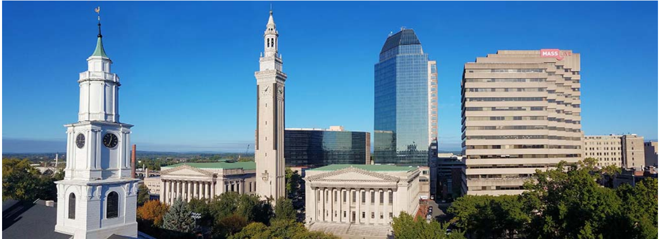
View of the Municipal Group of Buildings – Downtown Springfield, Massachusetts.
