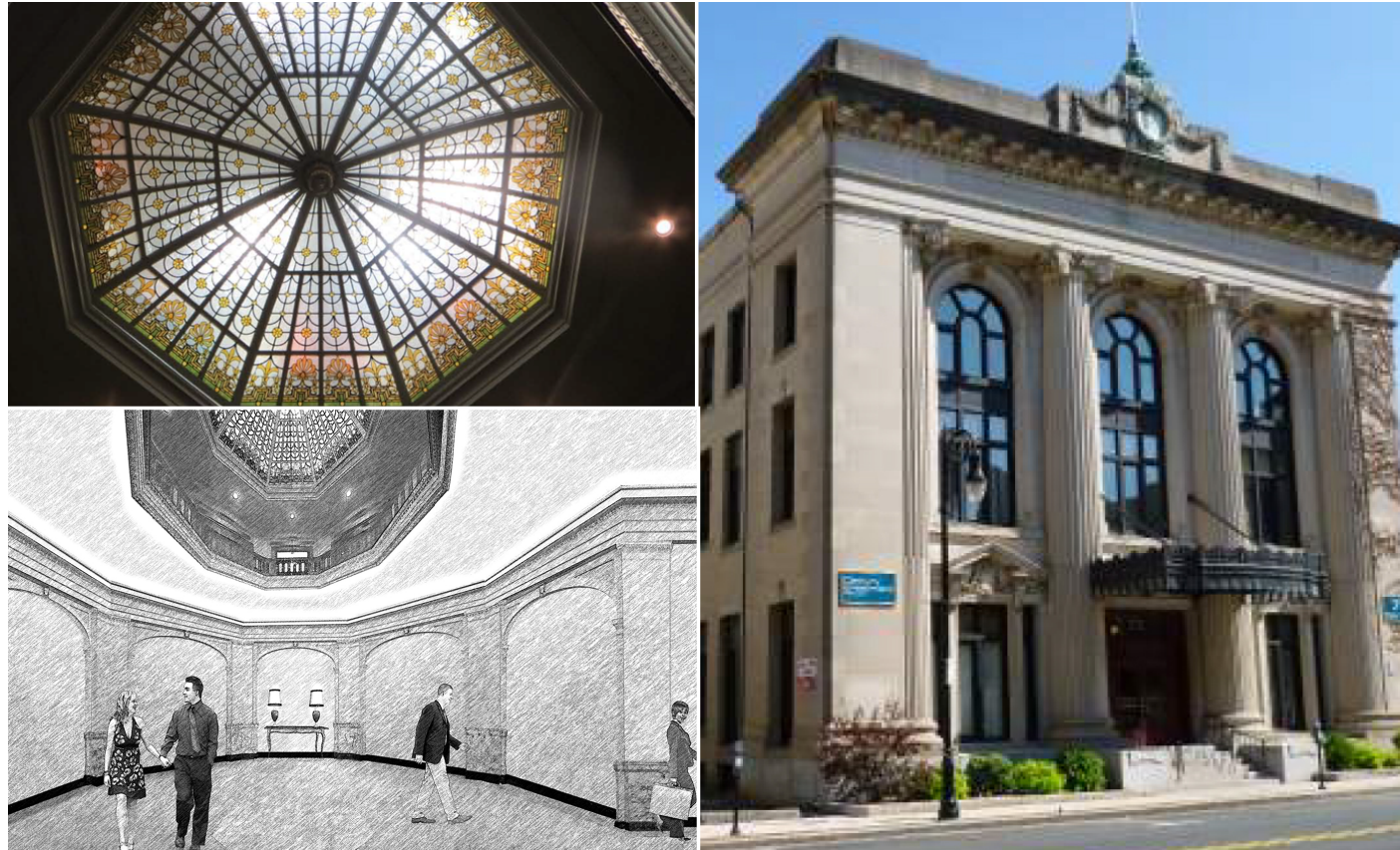
73 State Street Dome & Facade
