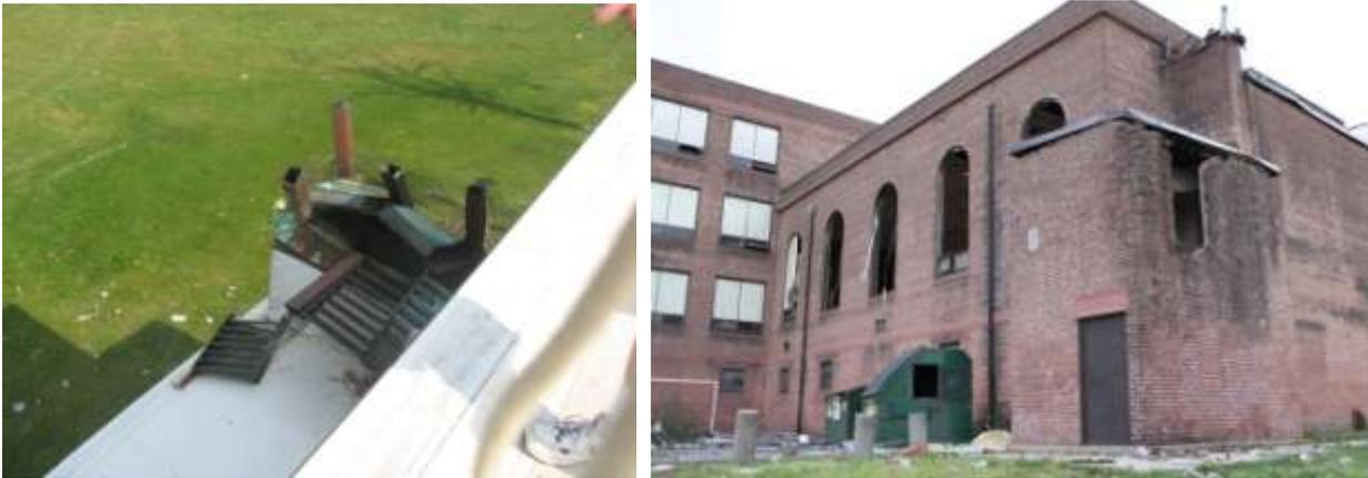
The main roof also suffered damage in several isolated areas caused by wind-blown debris which tore the membrane or was imbedded in the layers of insulation.
