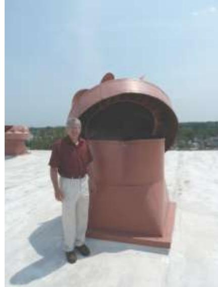
The rooftop ventilators, although re-installed, are damaged and probably not salvageable. Also rooftop condensing units appear to have been displaced and are probably damaged.
