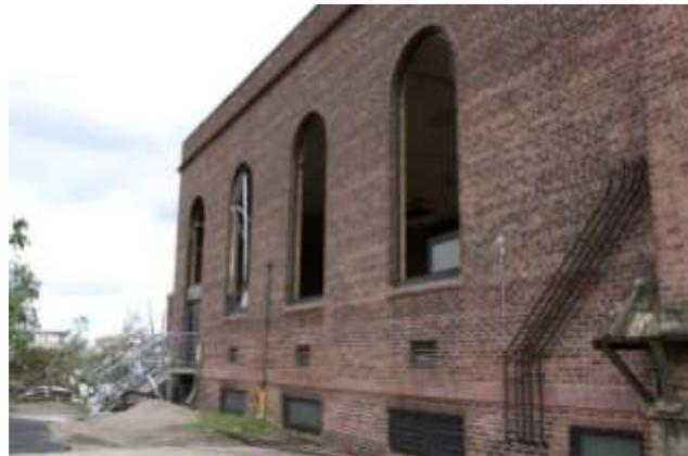
The brick parapets were blown off entirely at the south end of the main building and the lower portions of gym building had large sections of brick removed. These lower structures looked to be disconnected (not toothed-in) to the main gym structure and have been displaced.
