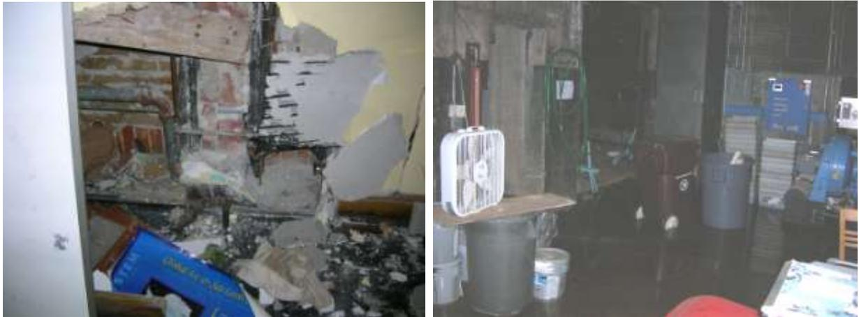
Since power was lost to the building during the storm, certain systems could not be observed to confirm their integrity. The loss of power did cause a failure of the basement sump pump which led to flooding of the basement; about 1"-2" of ground water was standing in the basement at the time of the professional team's visit.
