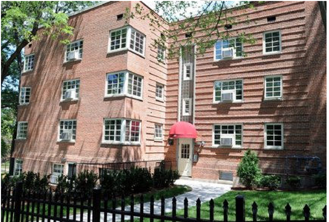
Forest Park Apartments HOME Rental Rehabilitation, 2010 Successful Renovation after Building Condemnation
