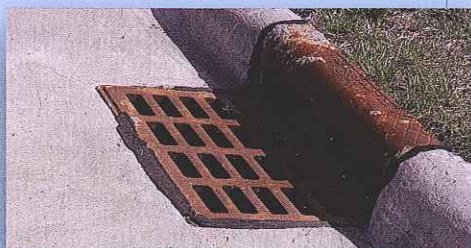
Storm Drain / Catch Basin
