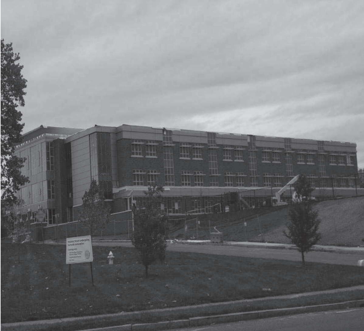
Construction of the new Elias Brookings Elementary School continues. To replace former school destroyed by the June 1, 2011 tornado.
