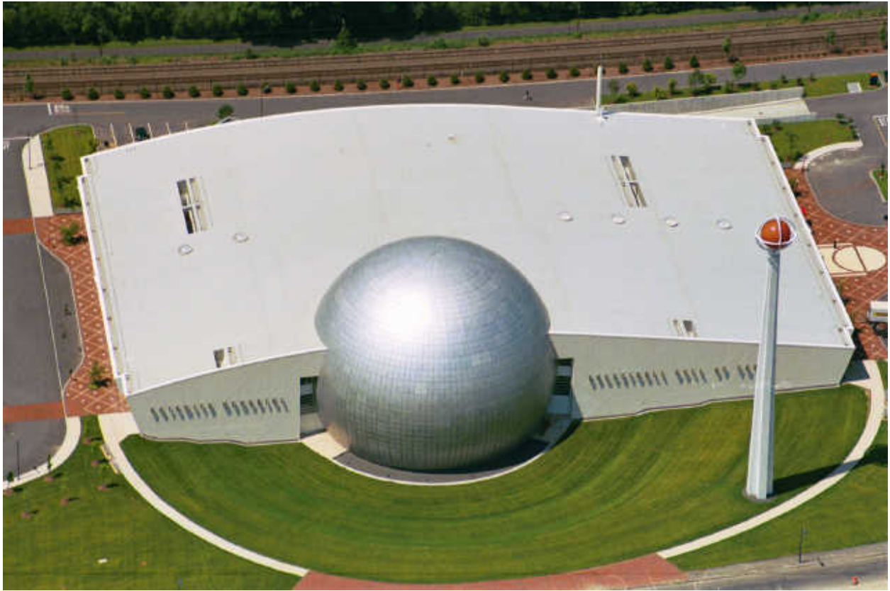
An aerial view of the Basketball Hall of Fame Located on the water front.
