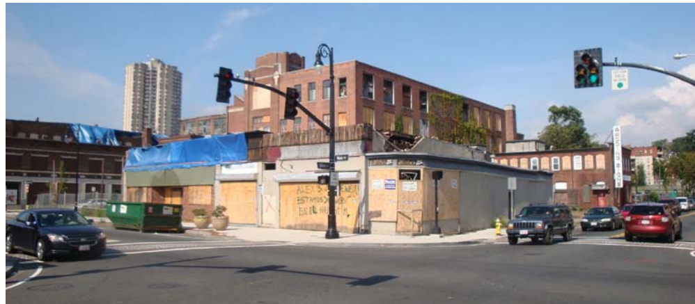
The eastern side of the Main and Union intersection was devastated by the tornado.
