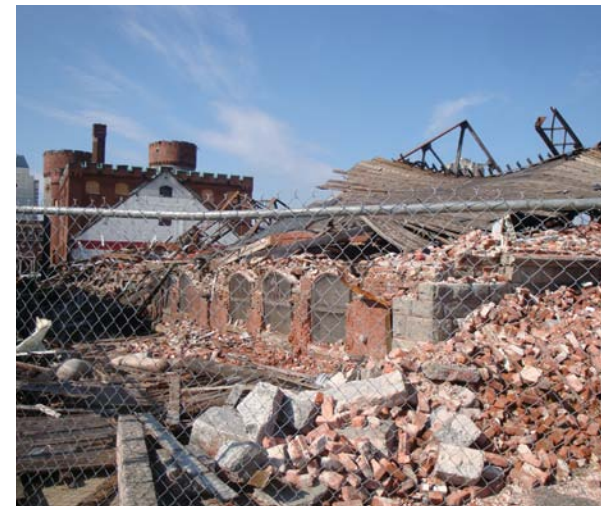
The Howard Street Armory, home of the South End Community Center, was significantly damaged by the tornado.
