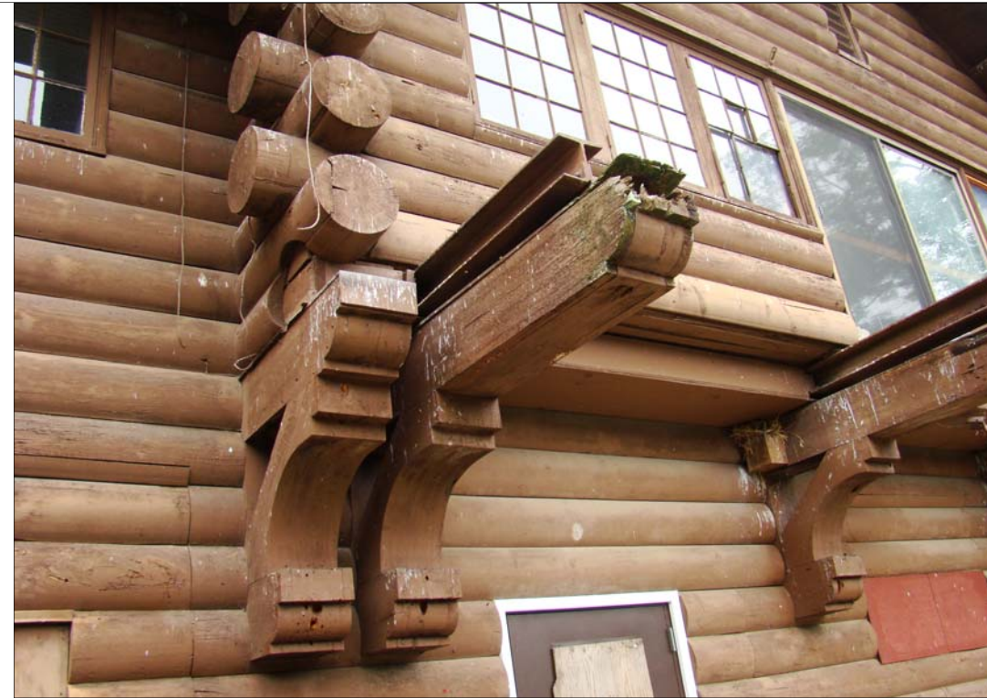
Picture #9 Close-up of architecture on south side
