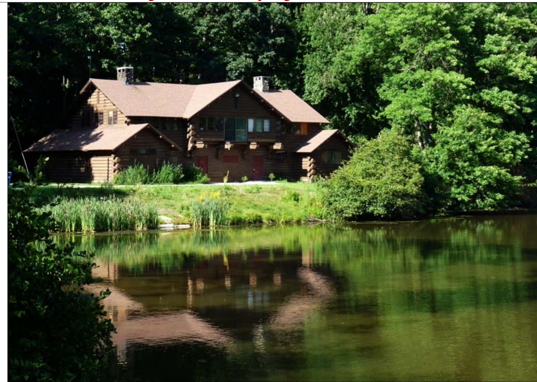
Picture #1: ECOS Center looking northeast across Porter Lake from Porter Lake Dam Road
