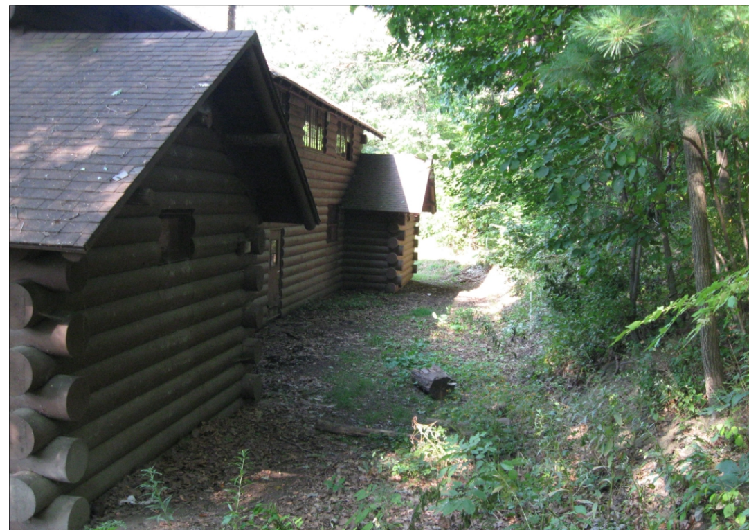
Picture #6: North side looking west/southwest
