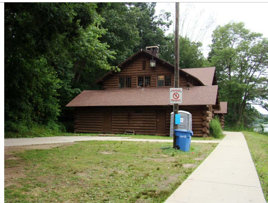
Picture #2: ECOS Center looking east from walkway off Porter Lake Dam Road
