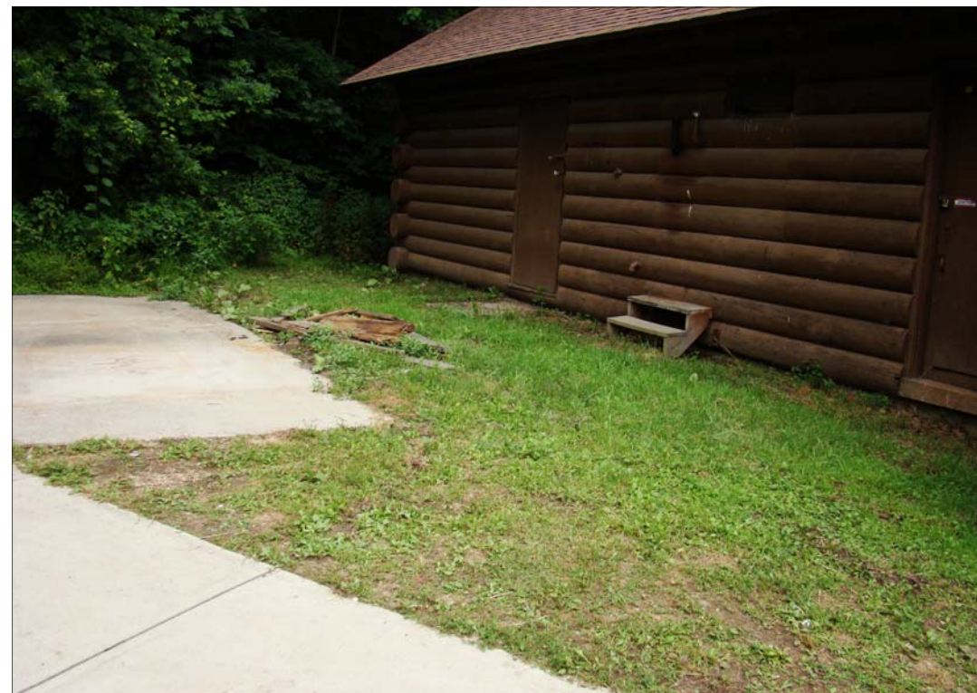
Picture #4: Close-up of west side looking northeast
