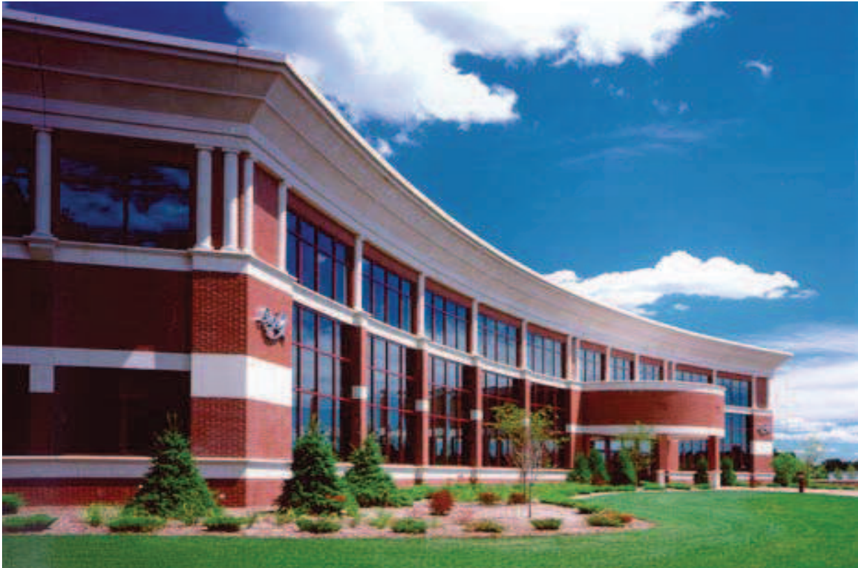
The headquarters of Big Y Supermarkets located on Roosevelt Avenue.
