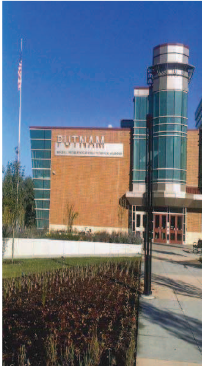
The newly renovated Putnam Vocational High School.
