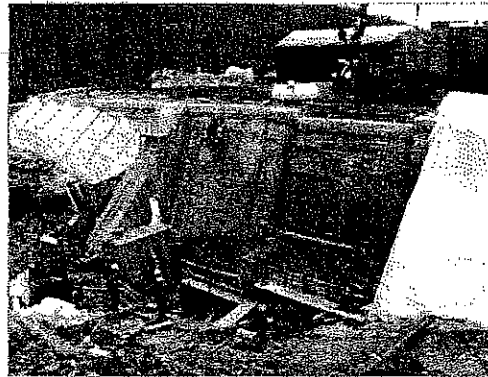
GZA engineers designed and inspected concrete repairs to the overflow sections of Lake Ladore Dam in Waymart, PA
