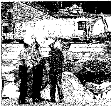
GZA regularly provides field engineering support services during the dam construction phase.
