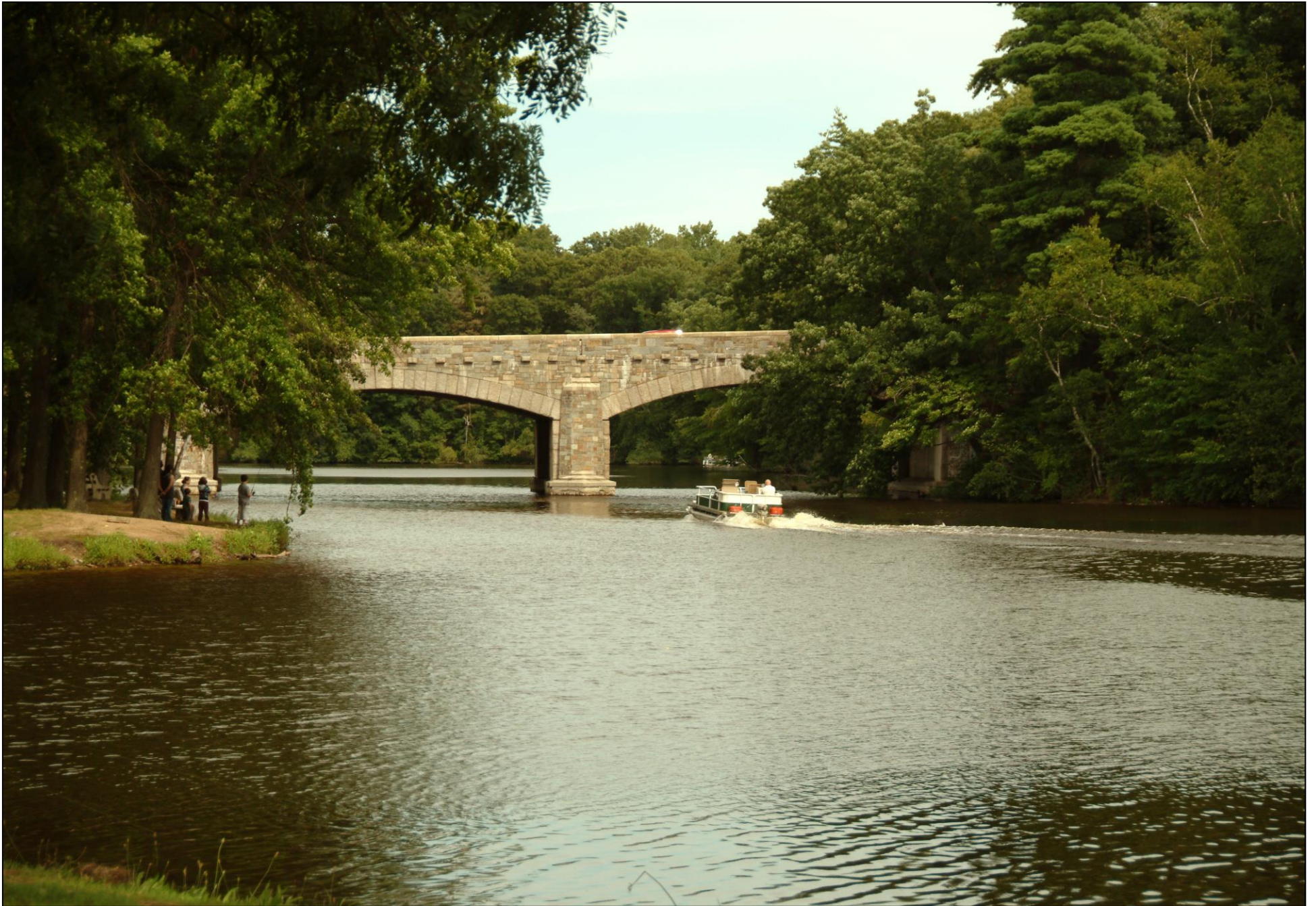
GENERAL EDWARDS BRIDGE FROM LAKE MASSASOIT
