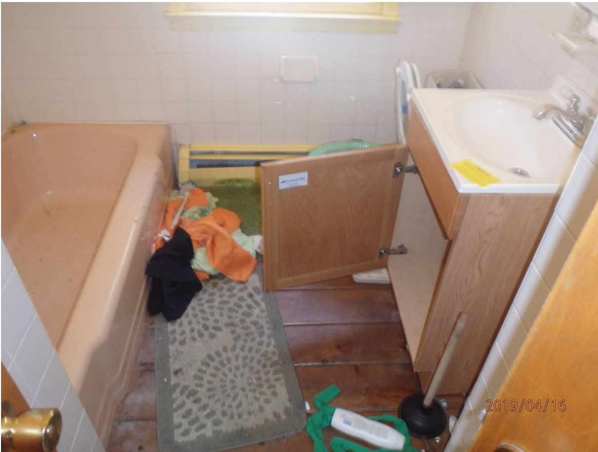
870 East St, Lenox MA – Before and after photos of bathroom.
