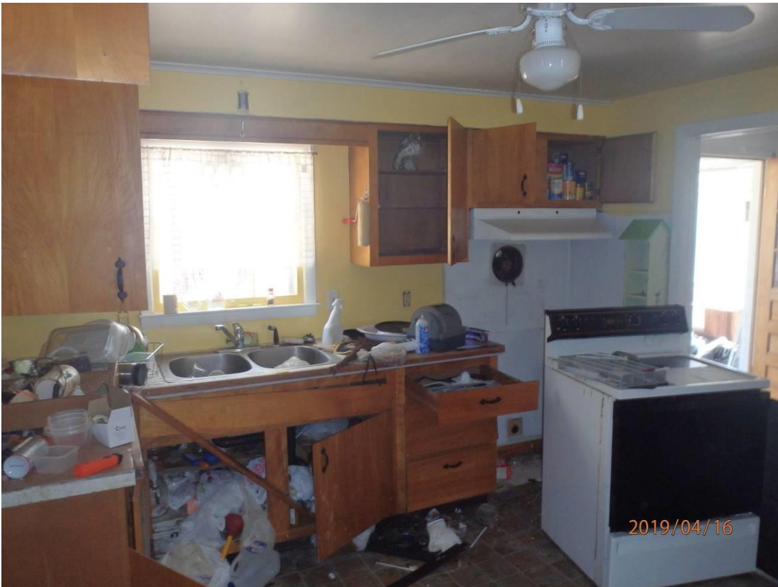
870 East St, Lenox MA – Before and after photos of kitchen.
