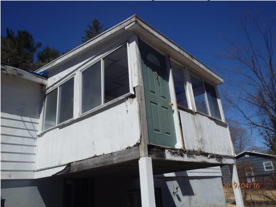
870 East St, Lenox MA – Before and after photo's or rear porch.
