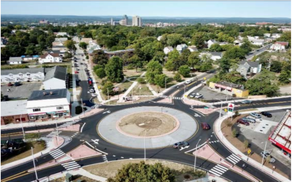
The redesigned intersection at Hancock, Alden, Walnut and Ashley Streets in Springfield – also known as Six Corners – on September 22, 2020. (Drone photo by Patrick Johnson / The Republican)
