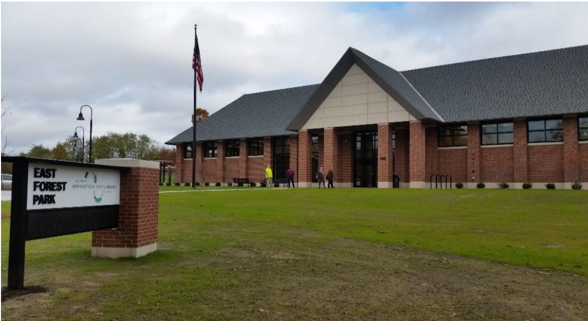
Newly built East Forest Park Library
