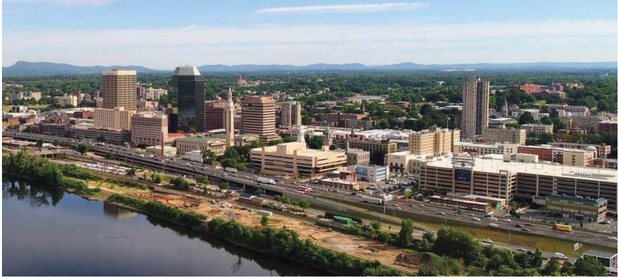
Riverfront Park, under construction 2018
