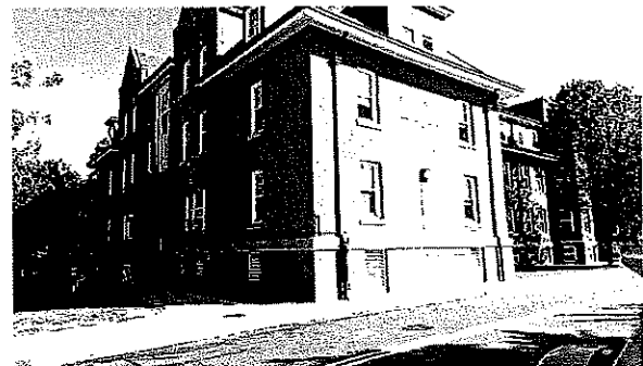
The building was inspected for interior concealed materials adjacent to the windows.
