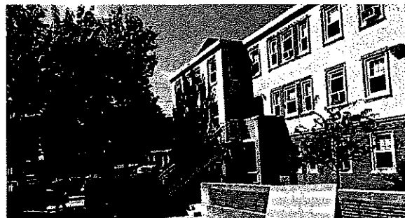
Large Scale Project - Renovation work includes replacement of the boiler plant, fire alarm system upgrades, as well as masonry restoration, landscaping, civil infrastructure, and development-wide site improvements.
