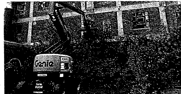
Hazardous Building Materials Investigation - Exterior building materials sampling at former Photech Facility.
