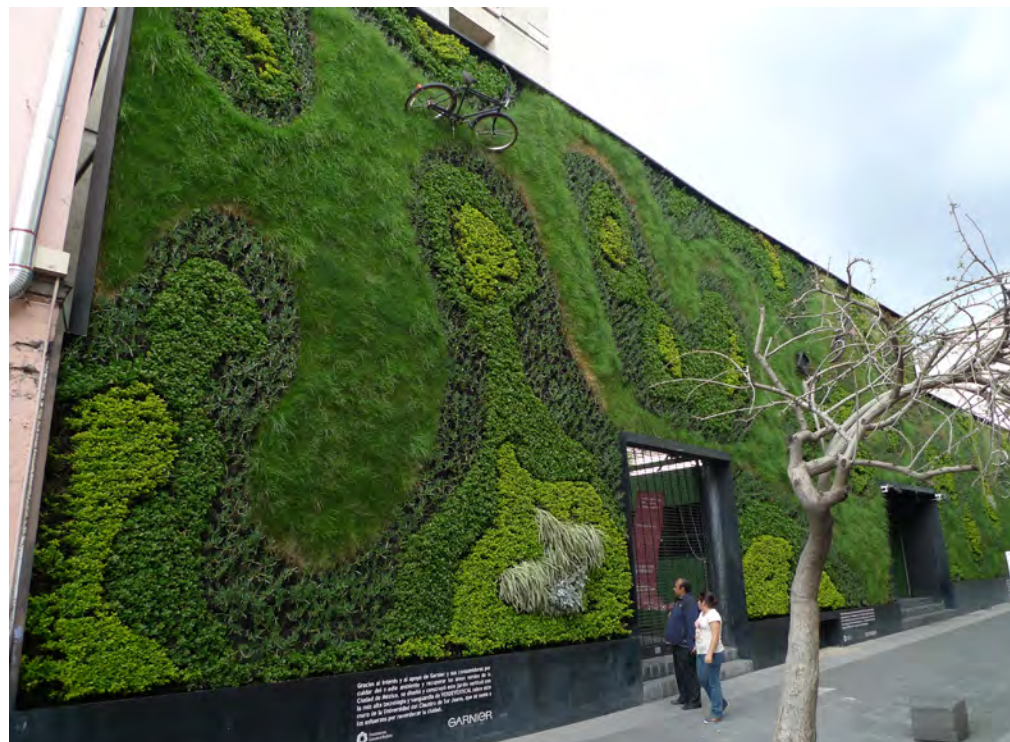
A green wall in Mexico City filters runoff and cools the urban environment, all while making an artistic statement.
