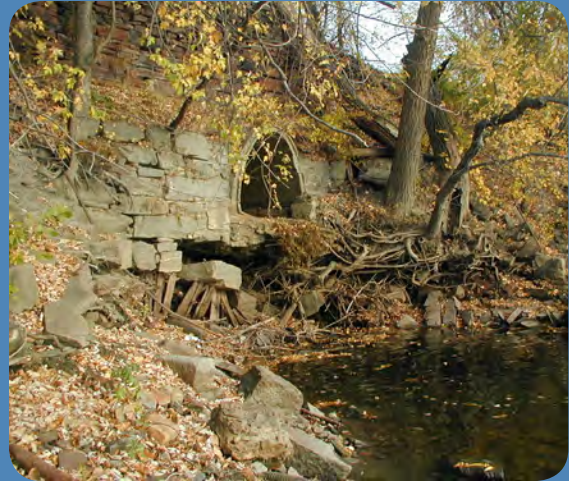
Springfield CSO Outfall Number 3.
