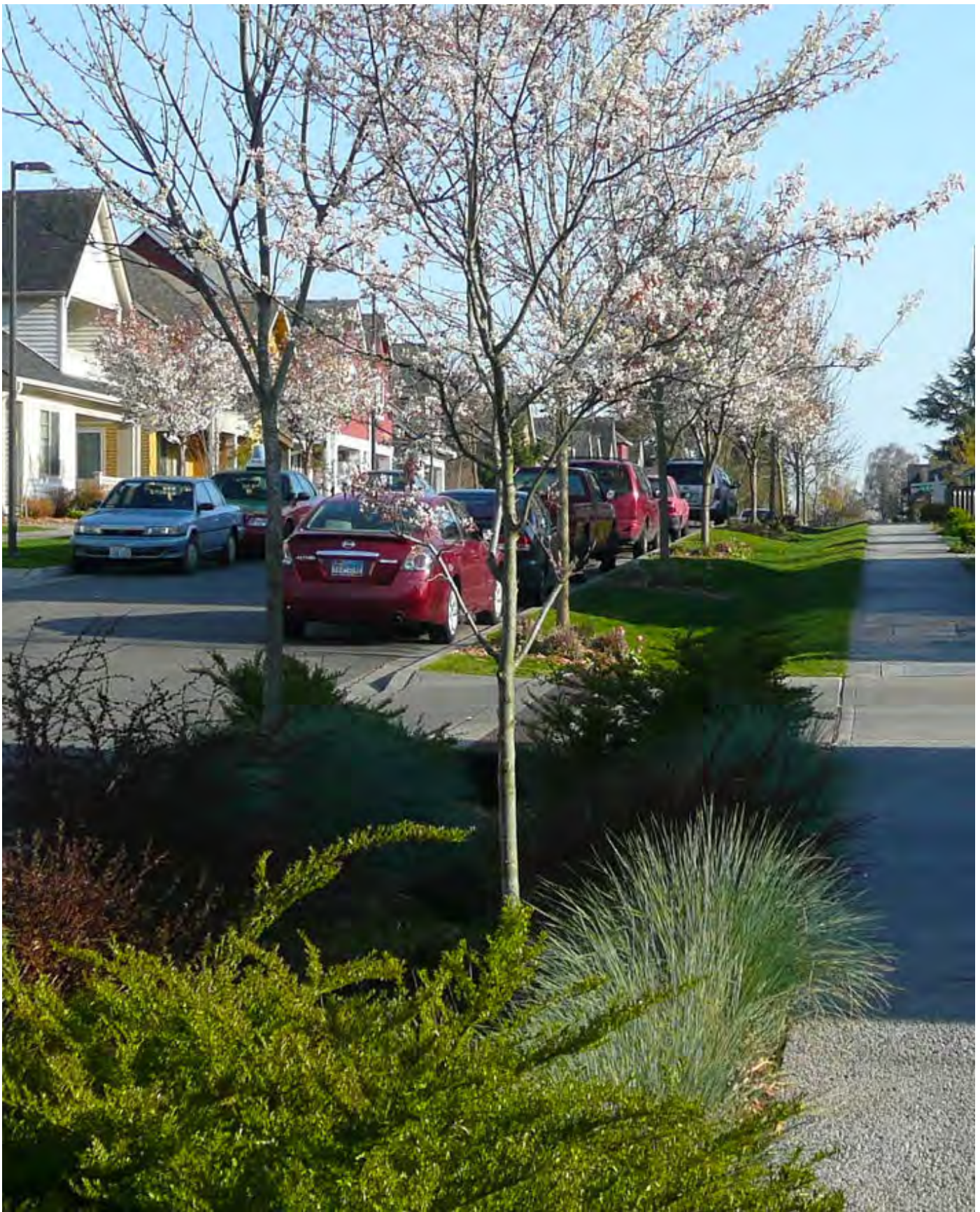
Green Streets can increase neighborhood aesthetics, such as this residential example in the High Point neighborhood of Seattle, WA.
