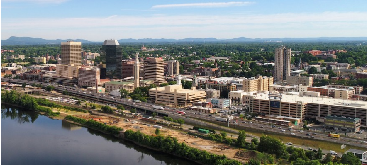
Riverfront Park, under construction 2018
