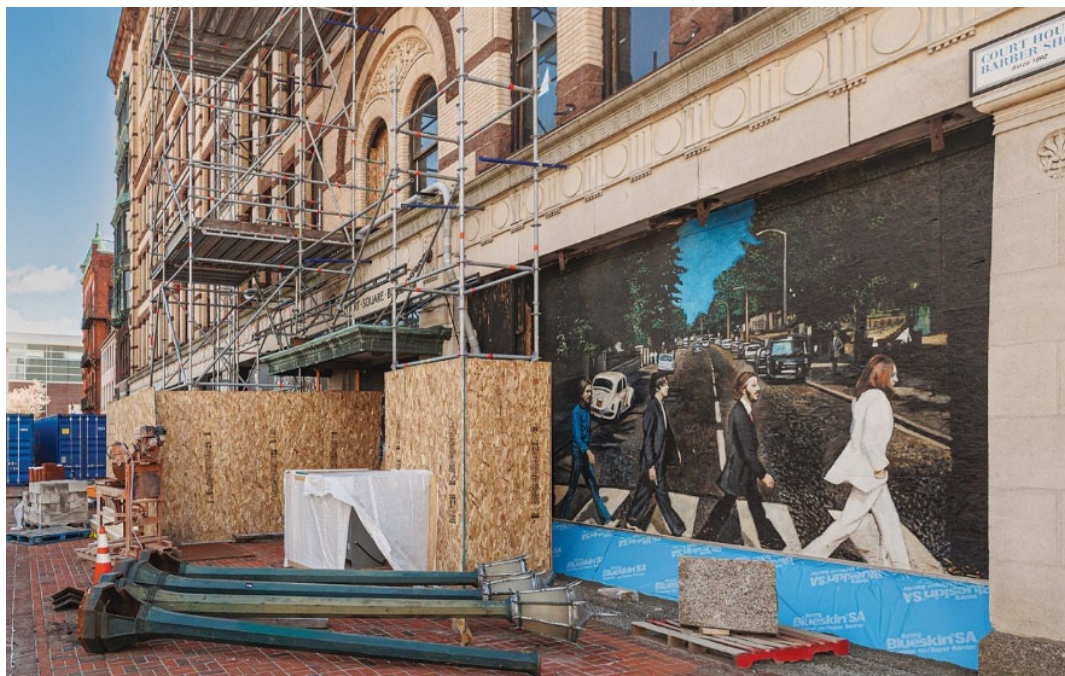
Historic Court Square Hotel is undergoing Renovation.
