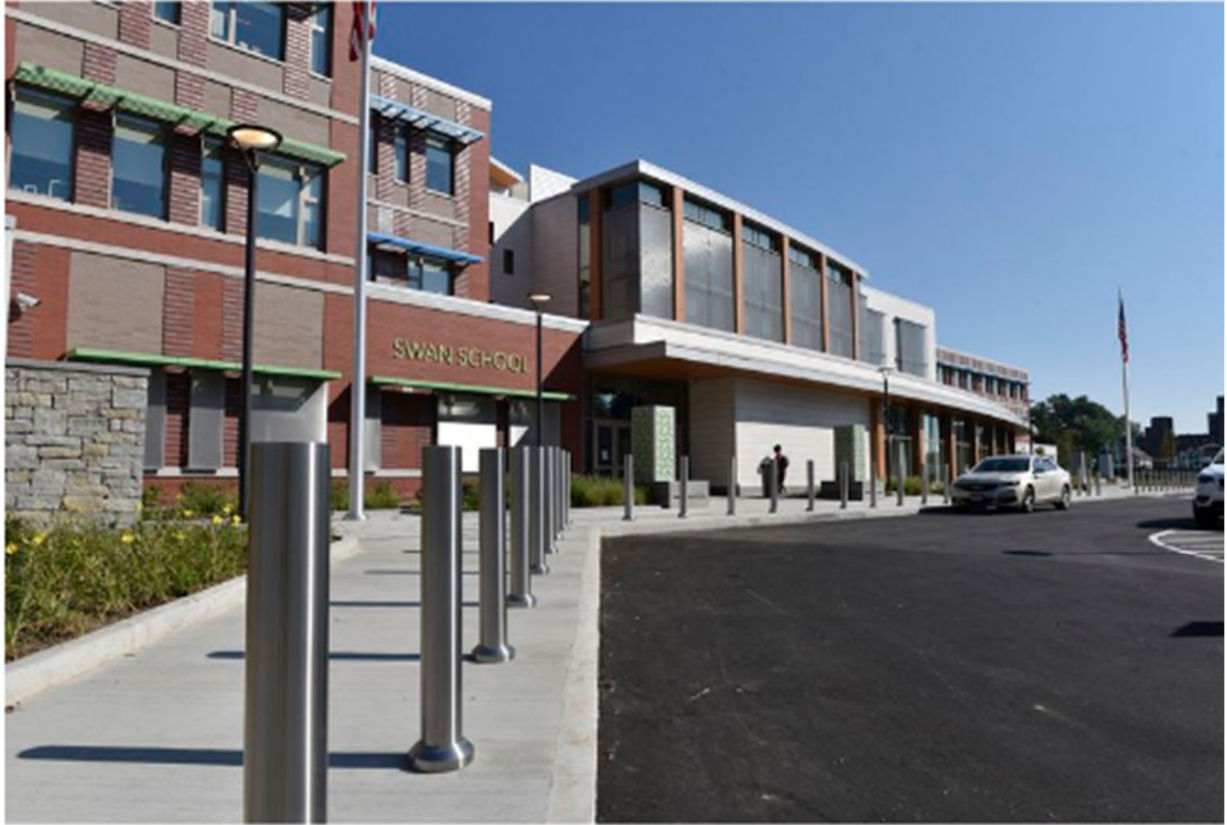
The new Deberry-Swan Elementary School in Springfield.
