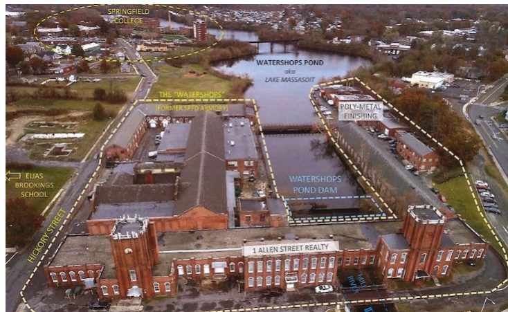
$2.5 million of improvements being done on Watershops Pond Dam.
