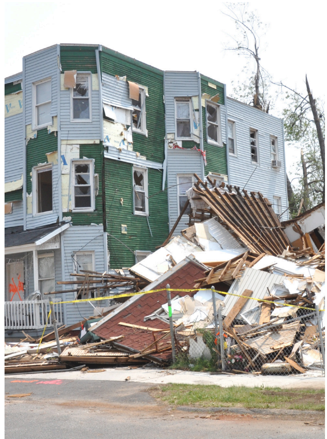
June 1, 2011 tornado damage
