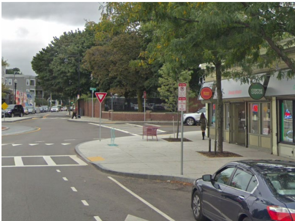
Figure 20. Example of permanent curb extension
