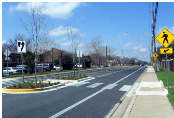
Figure 43. Example of pedestrian crossing at an uncontrolled location
