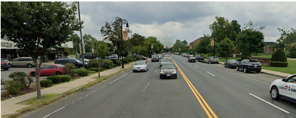
Figure 44. Opportunity to apply roadway conspicuity treatments along State Street
