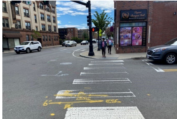
Figure 14. Example of faded crosswalks at Main/Fremont
