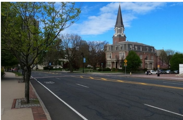
Figure 42. Example of a pedestrian crossing at an uncontrolled location on State Street
