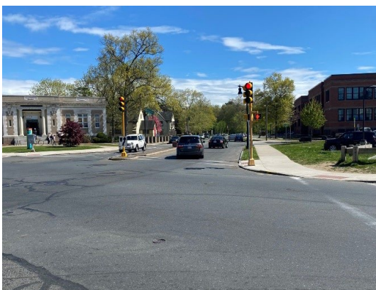
Figure 22. Opportunity for mast arm conversion at Oakland/Belmont
