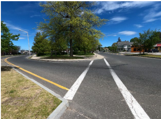
Figure 39. Opportunity to install high-visibility crosswalks at Saint James/Magazine
